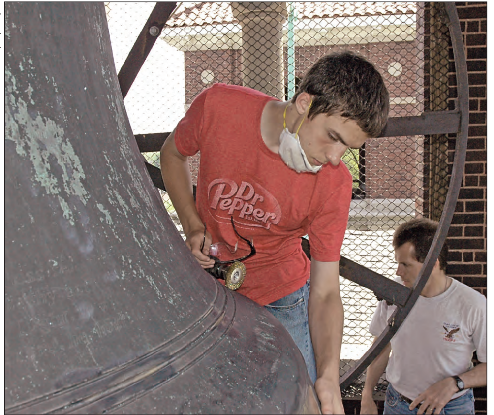
Our Lady of the Most Holy Rosary parishioners Ryne Friederick, left, and his father, Jerry, of Indianapolis begin restoration work on the bronze surface of the 7,000-pound San Salvador bell in the west belfry at the historic Italian church in Indianapolis on May 31. Ryne completed his Eagle Scout project in time for Holy Rosary Parish's 25th annual Italian Street Festival on June 13-14.
