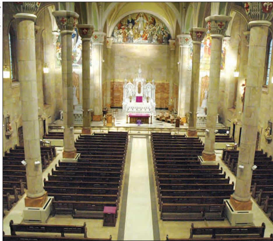
Above, St. Joseph Church in Jasper, Ind., in the Evansville Diocese, is the spiritual home for nearly 2,000 families in the area. The largest church building in Indiana when it was completed in 1880, it stands as a testament to the German-Catholic heritage of the region.
